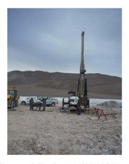
Photos 1 - Drilling Borehole PNN-VI-DW-01
