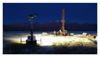
Photo 1 - Drilling Borehole PNN-SU-DW-01
