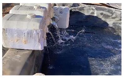
Photo 5-13 May - brine poured into prepared ponds with plastic liners
