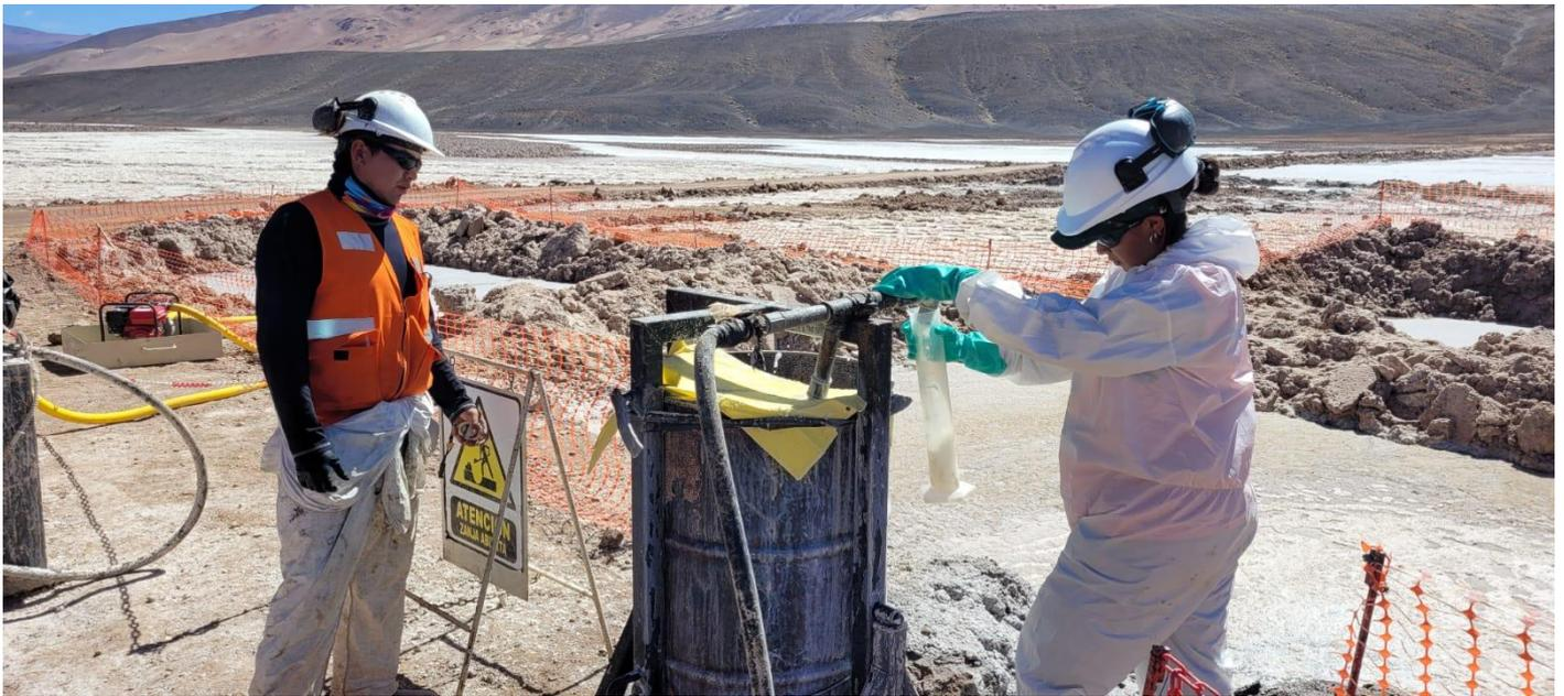
**Figure 4:** Brine sampling from drillhole PM23-IN-03 at the Incahuasi salar, Salta Lithium Project.
