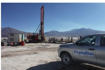
Drilling of the third borehole on Salar de Pular is at 110.5m. The borehole is planned to be drilled up to 350m.
