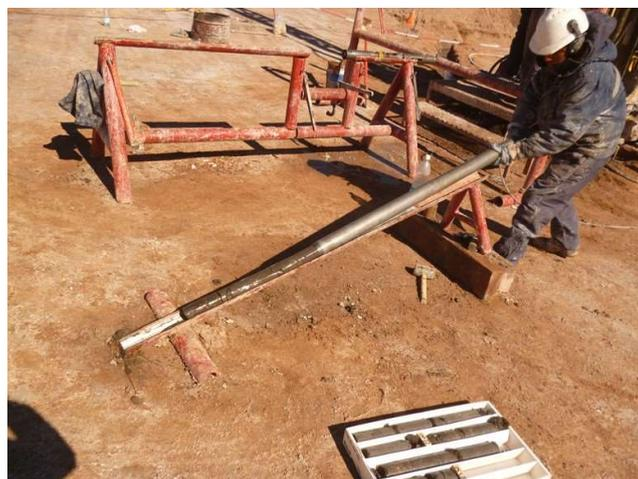
Photo 2 - Drill core extraction Borehole PNN-TP-DW-01
